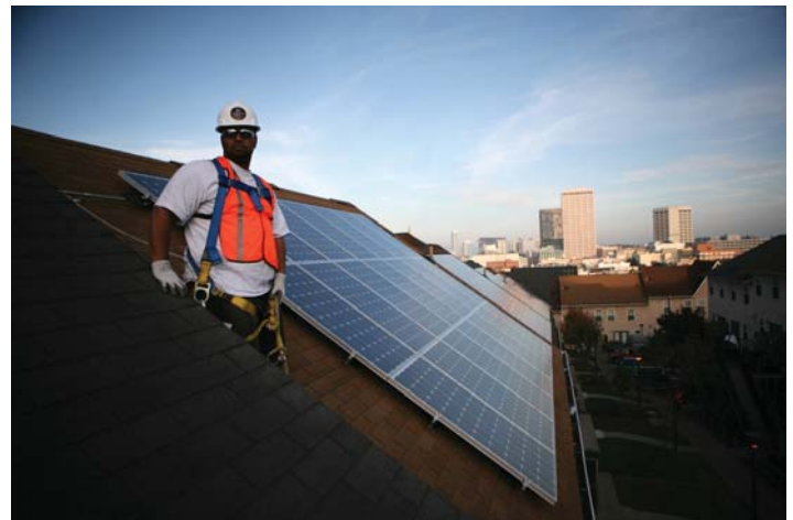
Photo Courtesy: Sunwheel Energy Partners
